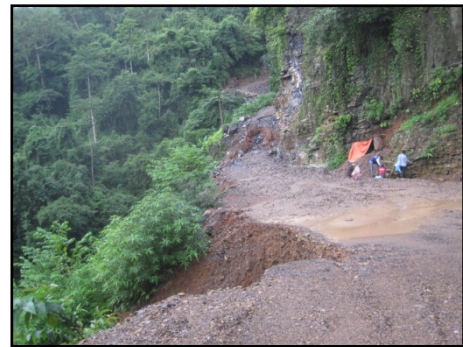
Figure 17 Debris flow in brecciated limestone of Moulmein Limestone (N16°49'15.4"E97°41'09.6", Facing - 280°)
