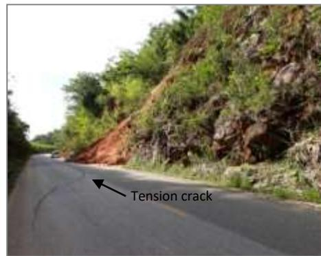
**Figure 7** Forming tension cracks indicate to occur circular failure.
