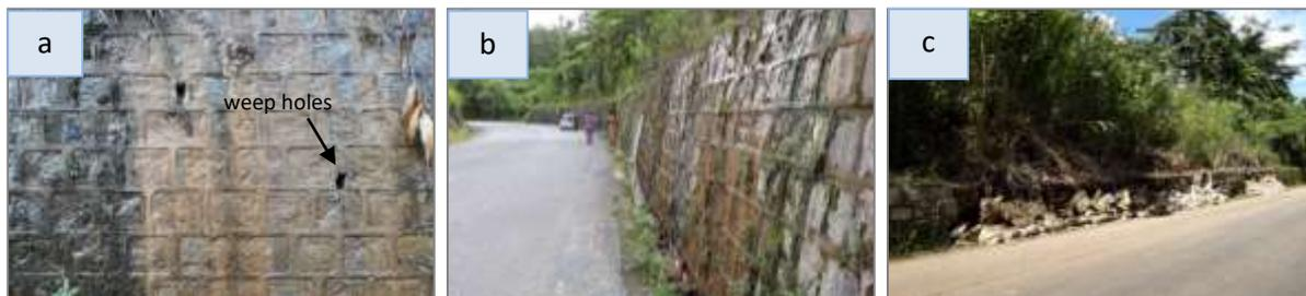
**Figure 9** Retaining walls, which have been constructed by granitoids, along the Mtitkyina-Kanpetii car road; (a) weep holes (b) wall without weep holes (c) damaged wall.
