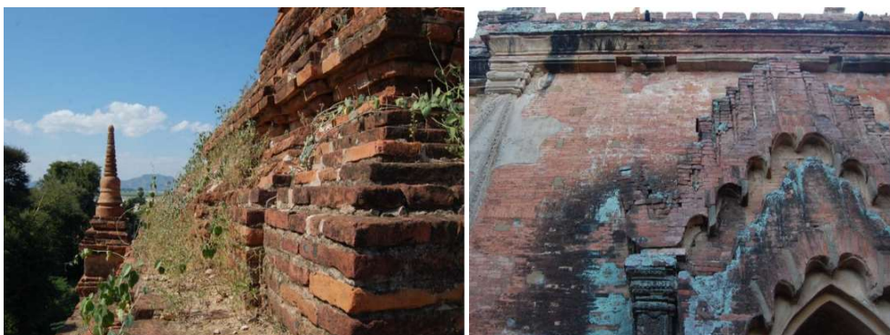
Figure (34) Damages Due to Vegetation and Microorganism
